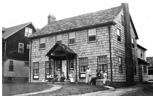
Figure xxvii: Architect/ builder Ray Hummer created typical side-by-side double 2928-30 E. Derbyshire Road as his family's home (files of Hummer, Lenore Weger, 1924)
