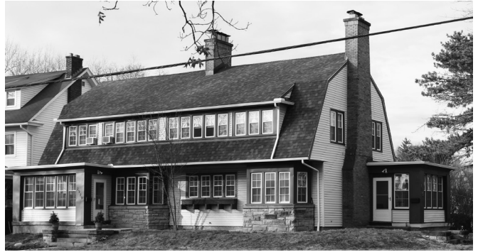
Figure xxxiii: 2929 Meadowbrook Blvd. depicts a gambrel-roofed variant to the Type 5 double. (Peskin, L.)
