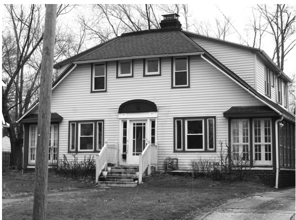
Figure xix: 3300 Dellwood Road is an unusual variation on a Type 3 double; it has a jerkinhead roof and large side dormers (Peskin, L.)
