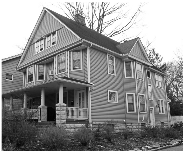
Figure xxvi: Pre-1909 home, 2264 Grandview Avenue, is a Type 3 double, though on the corner at Cecil Place. (Peskin, L.)
