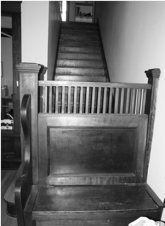
Figure xlii: built-in bench at 2332 Bellfield Avenue; stair rail serves as seat back (Peskin, L.)
