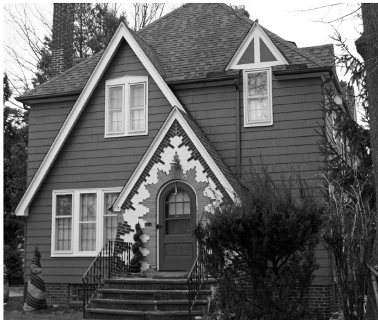
Figure li: The fanciful, two-colored brickwork on 3986 Bluestone Road's entry door surround exemplifies the Storybook Style interest of its builder, William Ingram (Peskin, L.).
