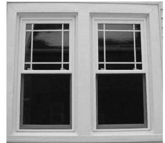
ABOVE: Figure lviii: Close-up of Wrightesque perimeter grid window at otherwise typical Type 1 triple, 3165 Meadowbrook Blvd (Owen, Chuck)
